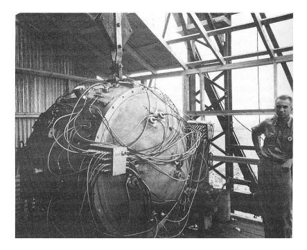
Here's the bomb on the tower. The cables run to our electric detonators. That's Norris Bradbury on the tower with it. It must have been pretty scary, for those who had to be on the tower that night, with lightning going on around them.
